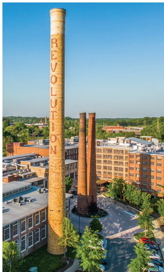
Revolution Mill's architectural features include large windows and three smokestacks.
